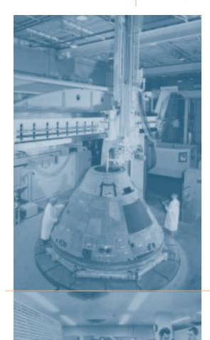
Run by an IBM System/360, a massive turret lathe shapes a heat shield for an Apollo spacecraft.
