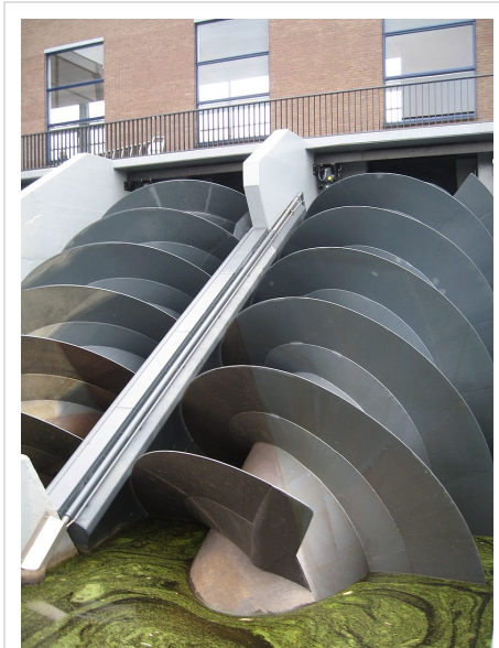
Archimedes' screw uses simple machines to lift liquids.
